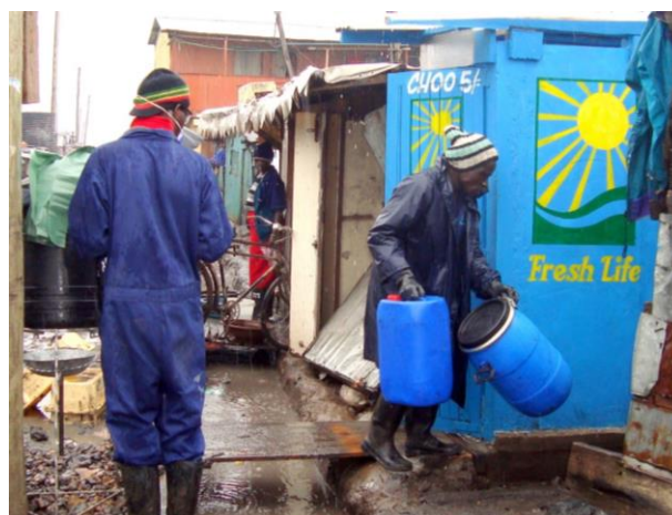
Workers remove the sealed portable containers that hold solid waste from a brightly colored Fresh Life Toilet in Nairobi.
